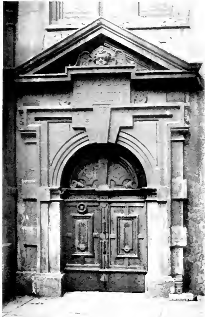
164. South Doorway, St Helen's, Bishopsgate.
